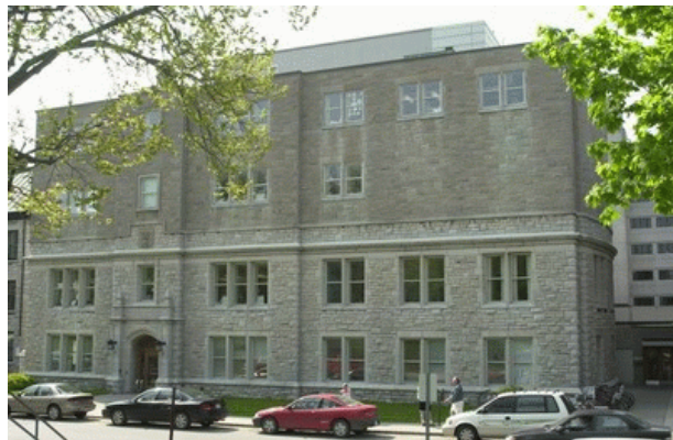
Looking southeast at Richardson Labs
